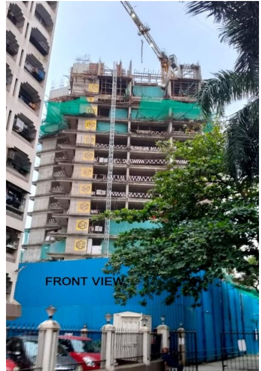
BUILDING FRONT VIEW
