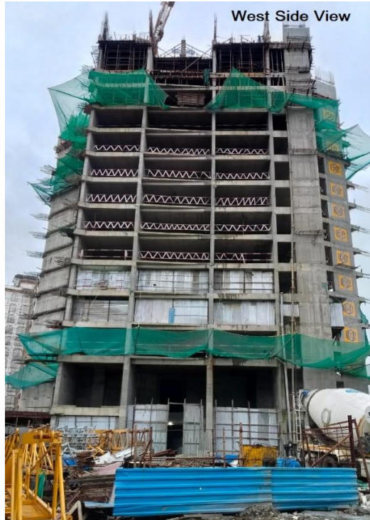
BUILDING WEST SIDE VIEW
